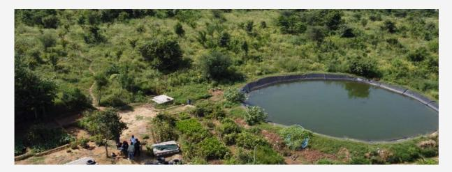
A pond has been created under Project Bhavnam for water harvesting and storing water for trees. In the rainy season, the water from rains is stored in the pond and is used to water trees in the Aravallis. During the non-rainy season, when all the water from the pond is used then water is pumped from the tube well post which it is stored in the pond and used to water trees planted on site. The pond rejuvenation initiative will **increase biodiversity** in the area.
