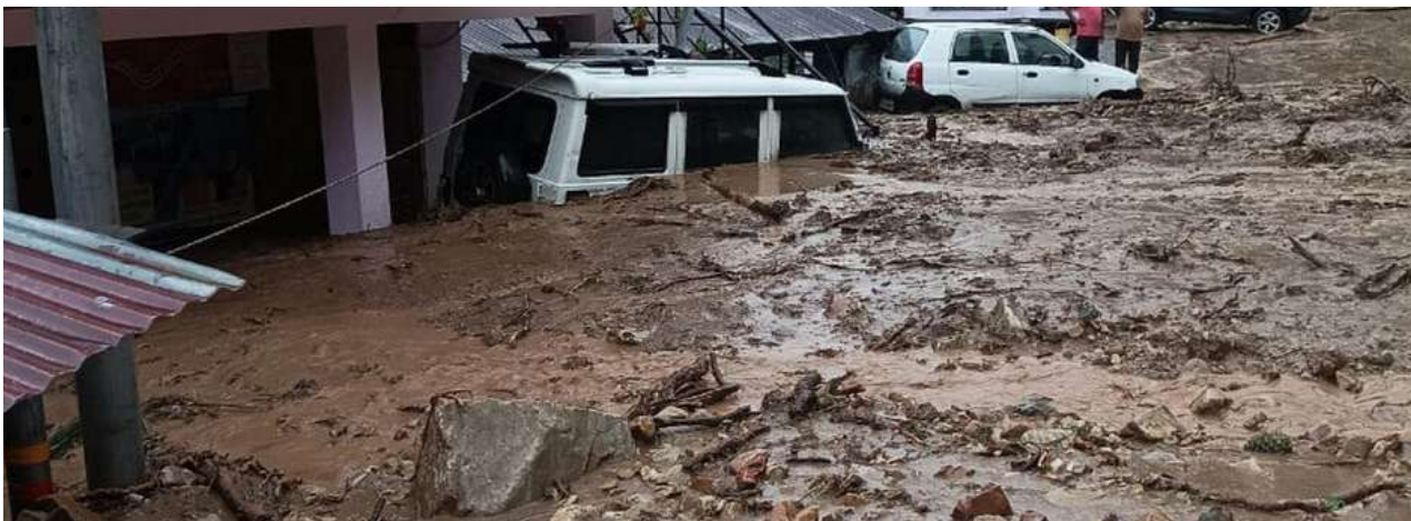
Flash floods after cloudbursts in Uttarkashi on 22 July 2023, causing damage to homes, vehicles, and roads
